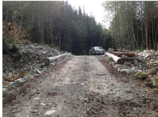
Approach from Right Bank when facing downstream
