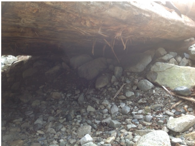
Left Bank Abutment when facing downstream
