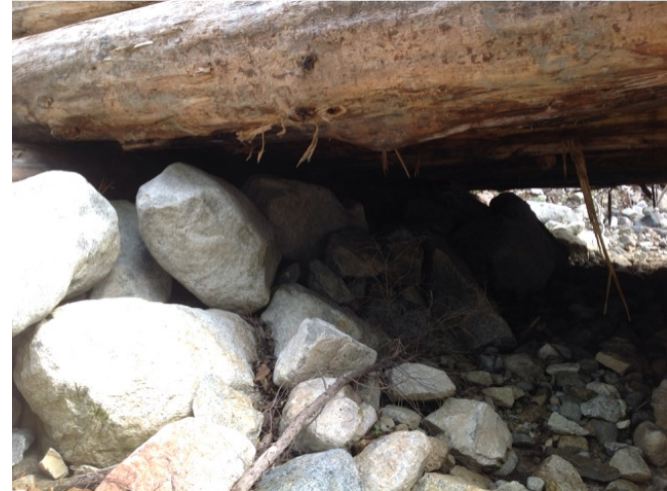
Right Bank Abutment when facing downstream
